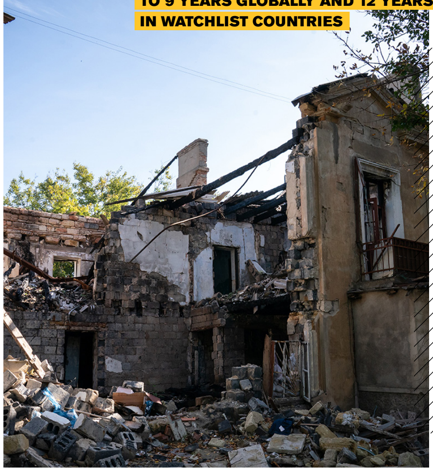
A residential building destroyed by a missile attack in Mykolaiv, Ukraine.
